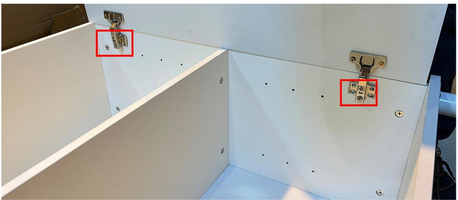
Gently flip the cabinet so the back is on the floor. The 4 small hole groups (4 per group) should face up. Attach doors 6 and 7. Use G to secure the other side of B.
