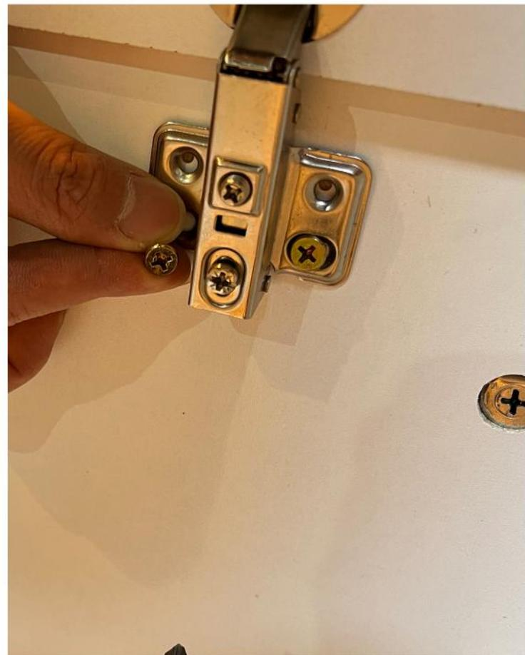
Install the two back screws first. Don't tighten yet — leave space to adjust. When all is correct, add and tighten all screws. You can adjust the door's height slightly—aim for even spacing rather than following the pre-drilled holes exactly.
