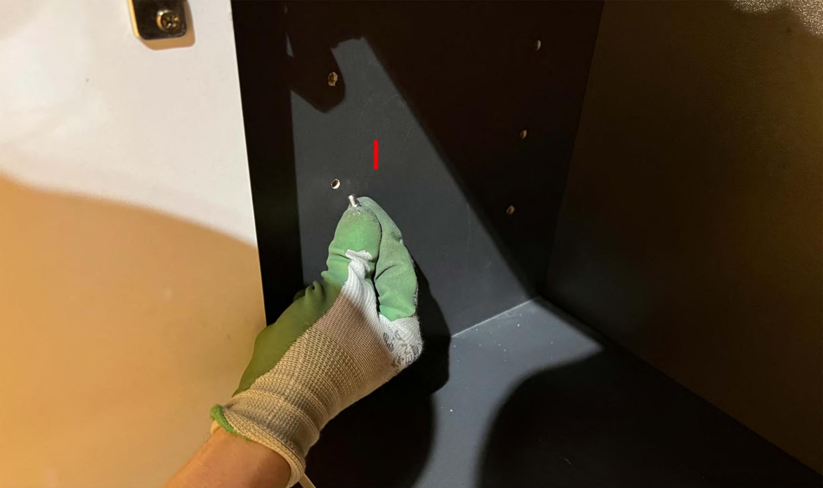
Install part 13 as needed. Insert part I into the matching pre-drilled hole on the appropriate side panel.
