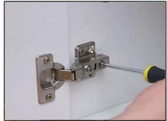
As shown in the figure, loosen the screw that the screwdriver points to, push the door panel in or pull it out, and then tighten it to solve the above problem.
