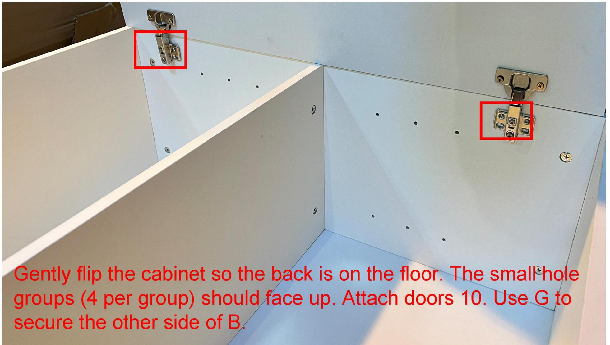
Gently flip the cabinet so the back is on the floor. The small hole groups (4 per group) should face up. Attach doors 10. Use G to secure the other side of B.
