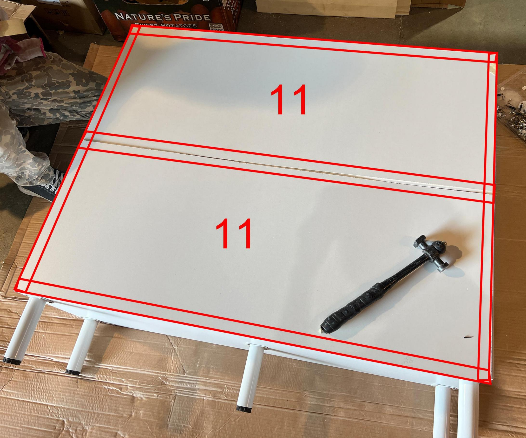
Place 11 (the back panel) in the correct position, fully covering the back side of the cabinet. Make sure to leave enough space along the edges for proper fastening by H. 11 x 2 should be installed using the same procedure. (Hammer not included.)
